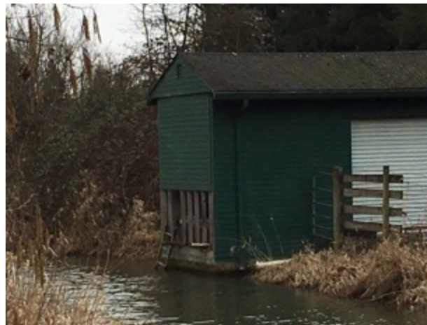
Pond facing side of pumphouse
