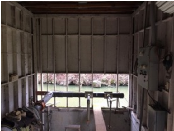
Wall facing the pond from inside
